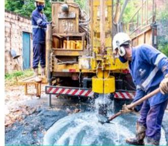
Drilled and reactivated wells
