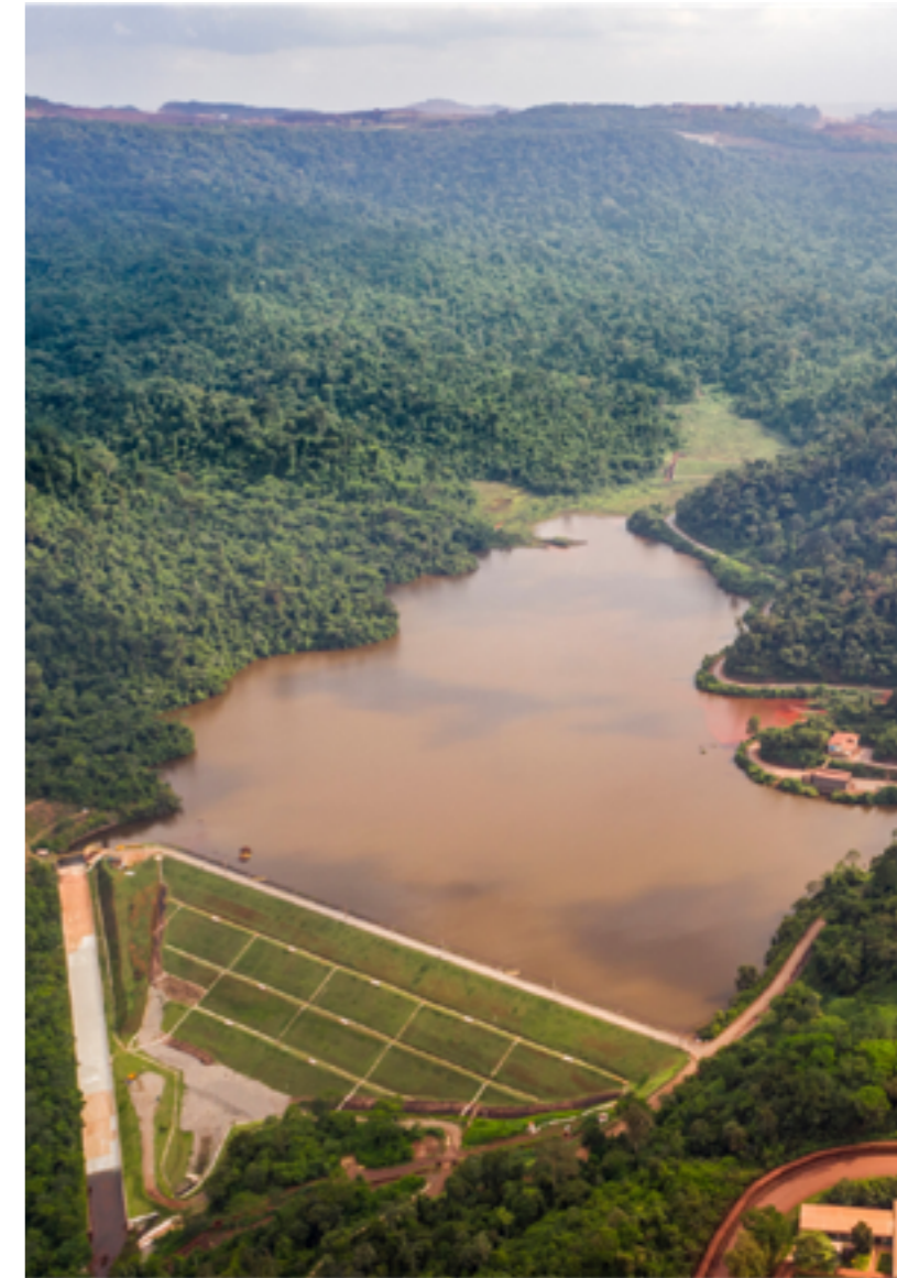
Serra Norte Dam, Carajás (PA) Photo: Ricardo Teles
