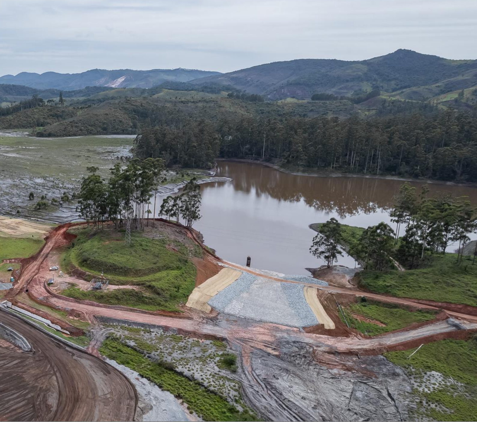
5 Pontal dike decharacterization works were concluded in December 2021
