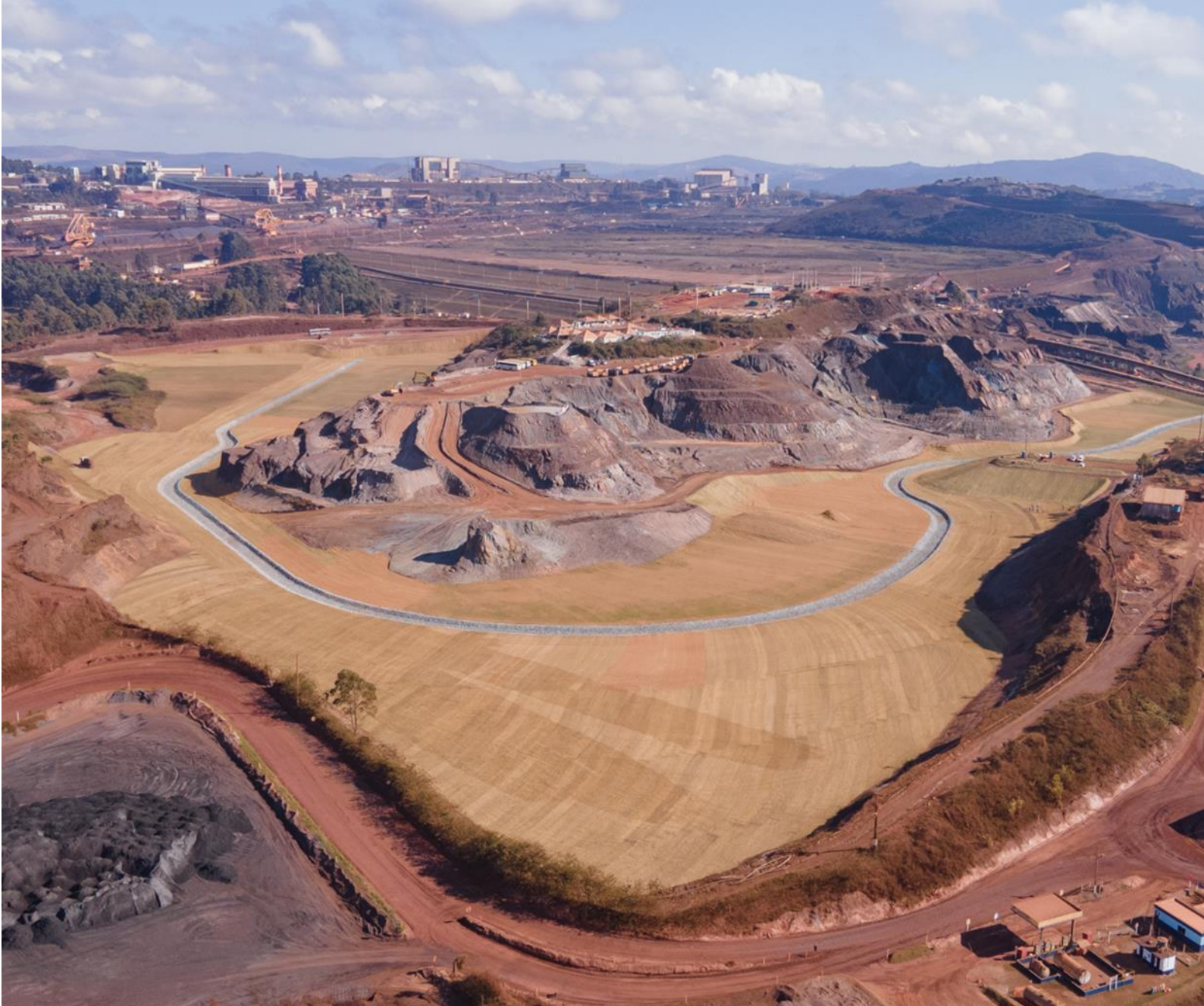
Fernandinho dam decharacterization works concluded in July 2021
