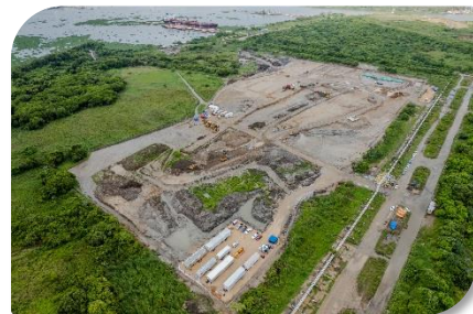
Aerial photo of construction site – Sep/22
