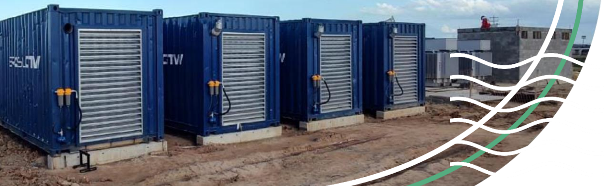
Gas to wire power generation system in the final stage of commissioning | Macau Cluster
