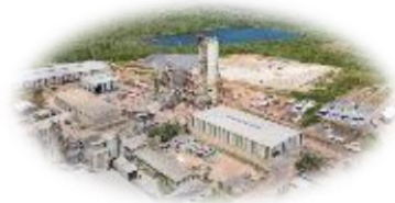
Pecém plant, Brazil
