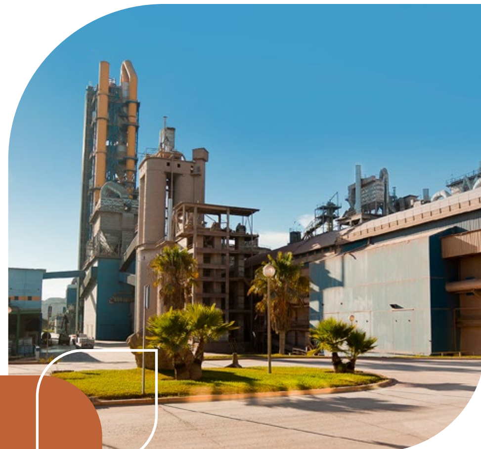
Málaga plant, Spain.
