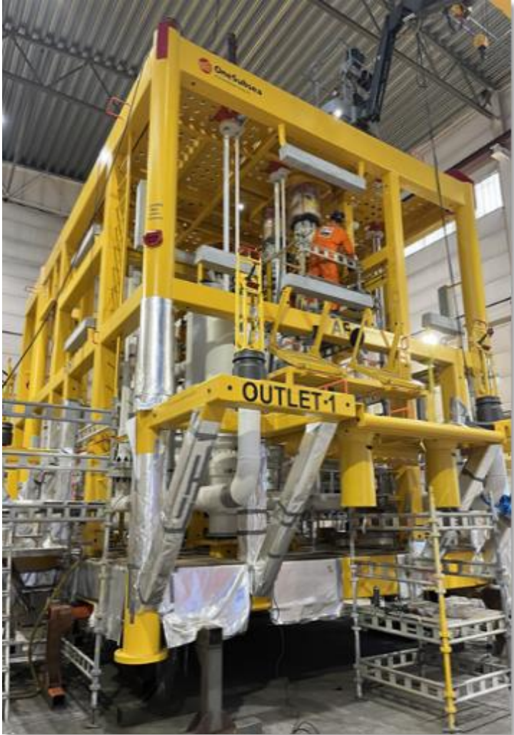
MPP skid completion for installation in Atlanta
