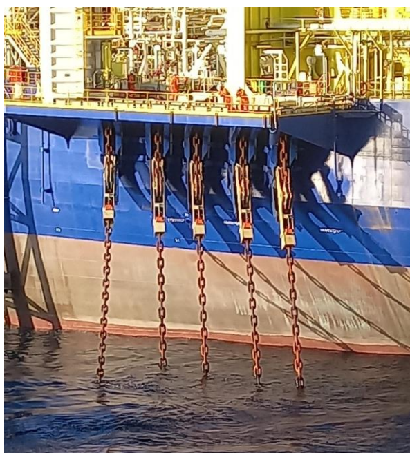
FPSO Atlanta anchoring installation in final phase
