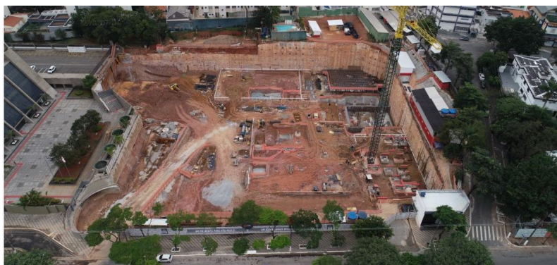
Picture of EZ Infinity's construction site
