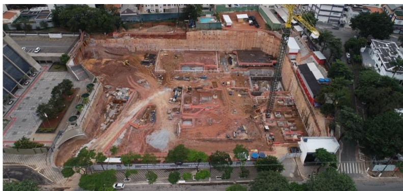
Picture of EZ Infinity's construction site
