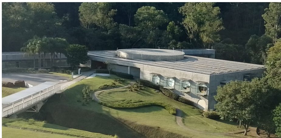
The roof of the NAN (Natura Learning Center) in Cajamar (SP) is covered with solar panels.
