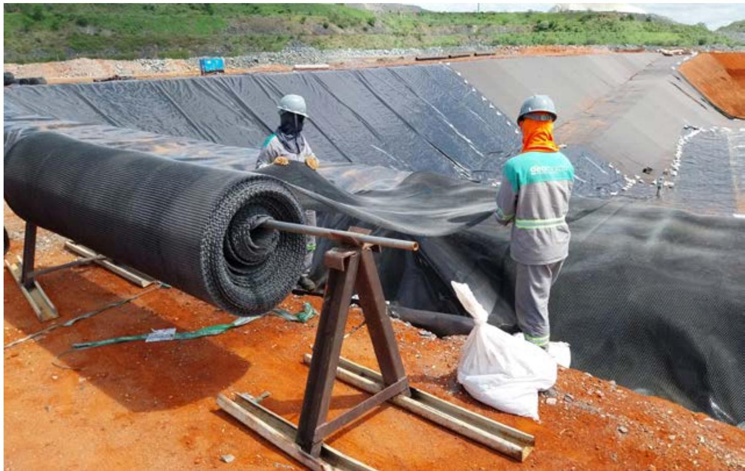
The design and project were based on extensive geotechnical investigations and the construction conformed with best-in-class engineering practices. The facilities are lined with two layers of geotextiles, providing excellent impermeability, preventing water infiltration, soil contamination and acid drainage. The groundwater quality is monitored in several points.
