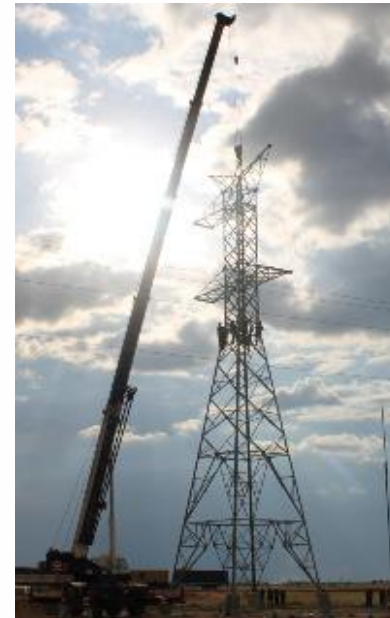
16 Transmission Line Towers concluded
