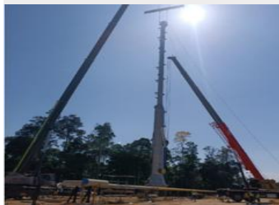
Flare and EMEDs assembly on the bases
