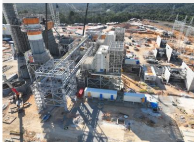
Receipt and start of assembly of maintenance and modularized pipe racks
