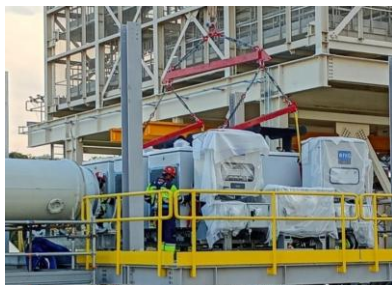
TPP: Main circuit breaker positioning (GT11 GCB)
