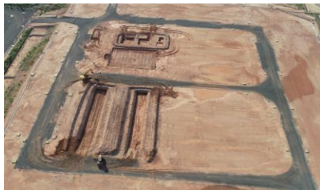
Start of Civil Works
