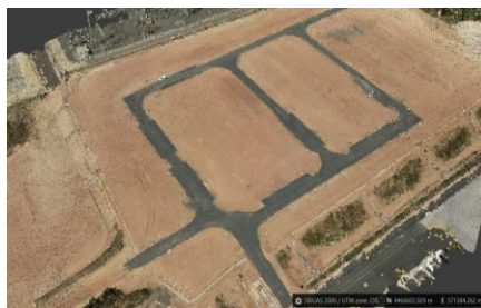
Completion of earthworks and access roads
