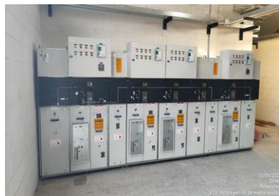
Water Intake System: Start of electrical panel assembly at the substation
