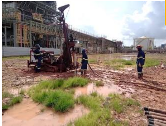
Pipe setting for cross hole test
