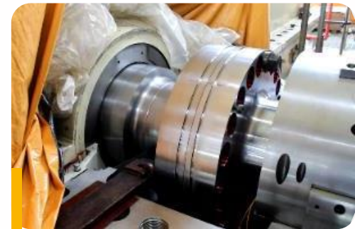
Start of turbine alignment
