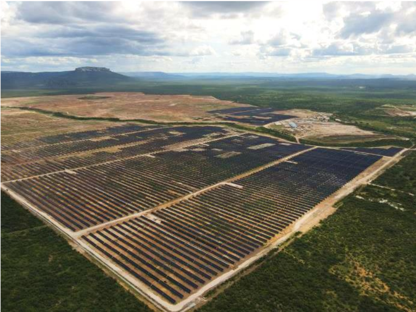
Assembly of modules
