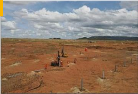
Drilling and nailing of piles
