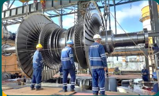
Steam turbine: last removal of the rotor for boroscopy and final cleaning
