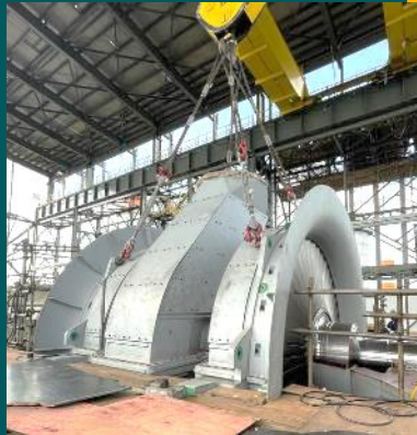
Definitive closing of the steam turbine
