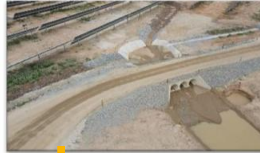
Digging of drainage channels and laying of low voltage cables
