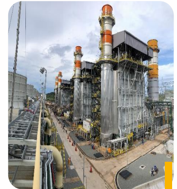
Completion of Sigma Clean of all boilers at Parnaíba V
