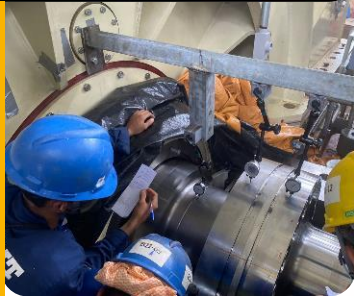
Turbine final alignment and Runout of steam turbine
