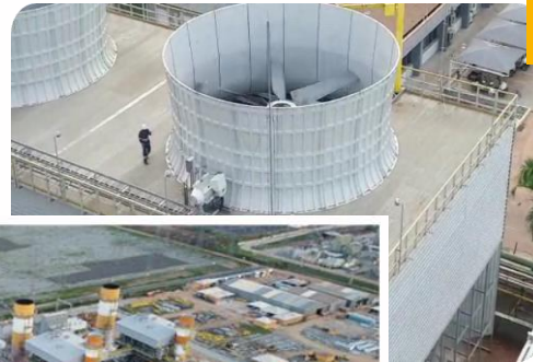
Completion of cooling tower commissioning
