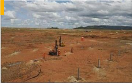
Drilling and nailing of piles
