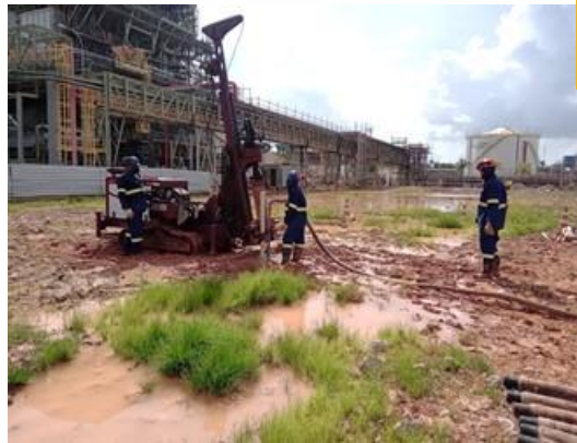
Pipe setting for cross hole test
