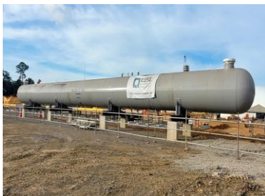
Positioning of slug catcher at the base
