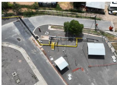
PTU – Start of cold commissioning
