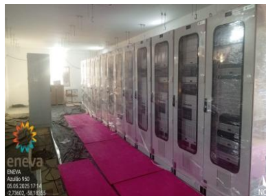
Assembly of SPCS panels
