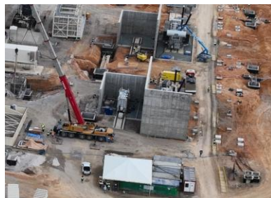
GTG11 – Positioning of Auxiliary Transf. 11BBT
