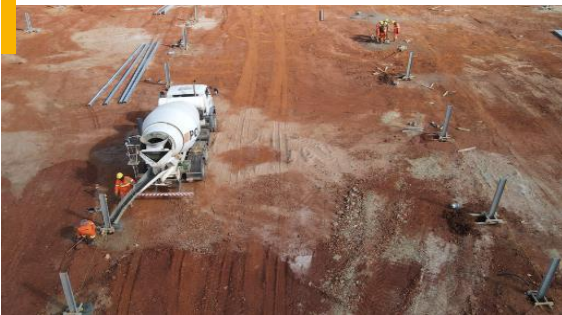
Drilling and nailing of piles
