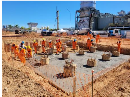
Foundation of the turbine base
