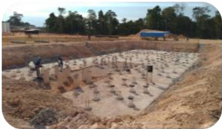
Condensate tank piles
