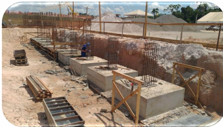
Concreting of the blocks - Isotank A axis
