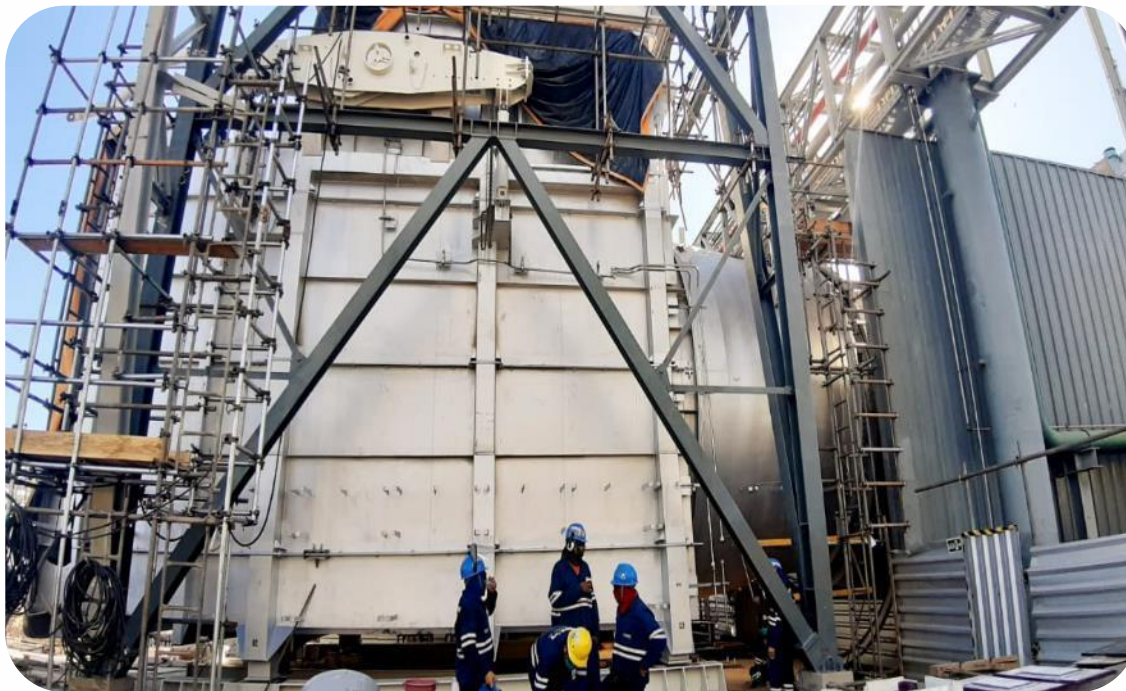
Installation of diverter 21 in the final position
