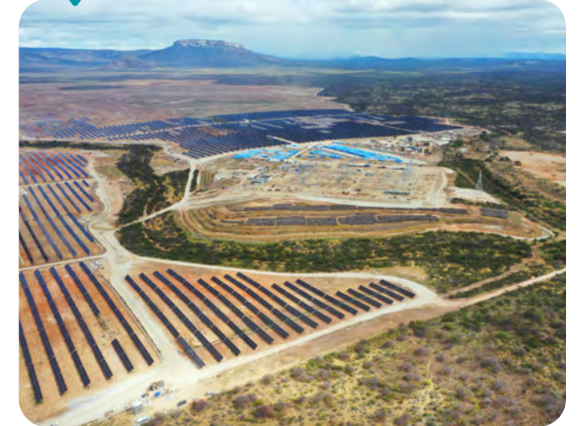
▼ Futura I Solar Complex
