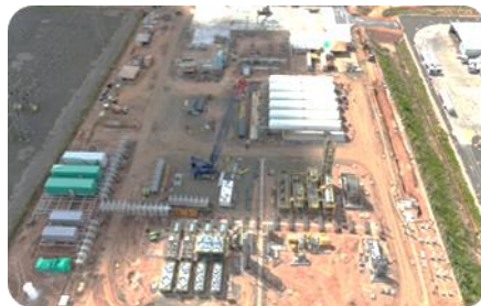
General Site View
