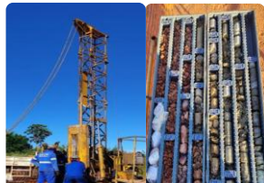
Soil boring and sample collection
