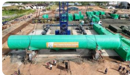
Unloading of Equipment onto Foundations
