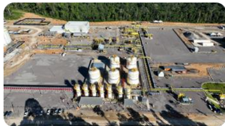
GTU: General aerial view
