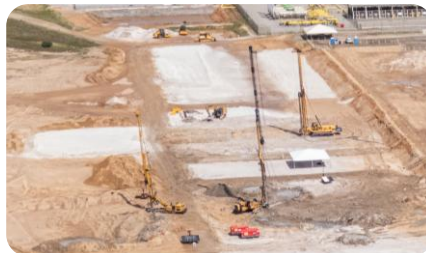
Piling Works Execution
