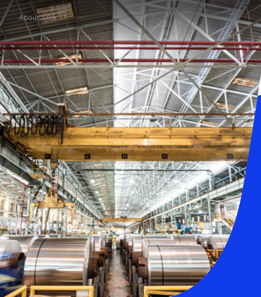
A rolling line at the Itapissuma rolling mill
