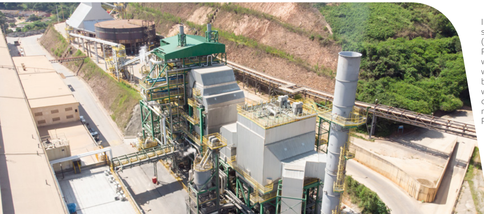
A biomass boiler to produce steam at the Alumina department
