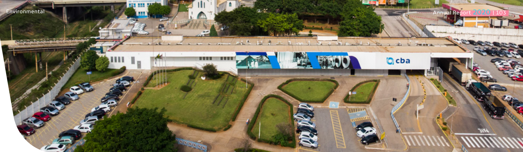
The facade of the Aluminio plant
