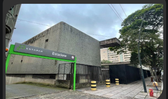
Duque Parking Building - RS
