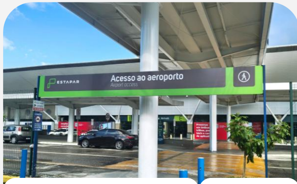
PARÁ Belém Airport
