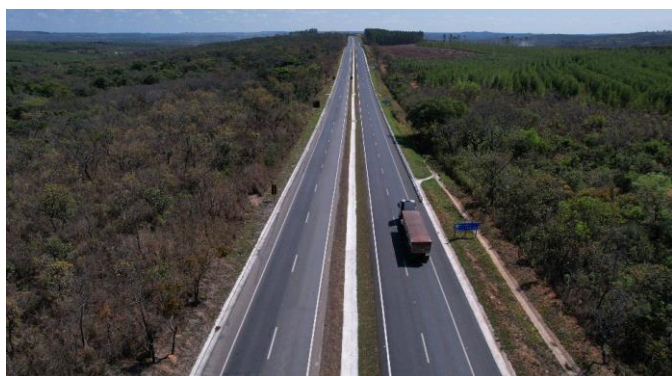
Eco135 Road widening
