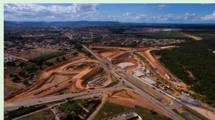
Eco135 - Construction work on the Montes Claros Ring Road
