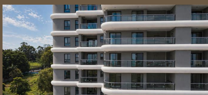
Paris Tower Façade
