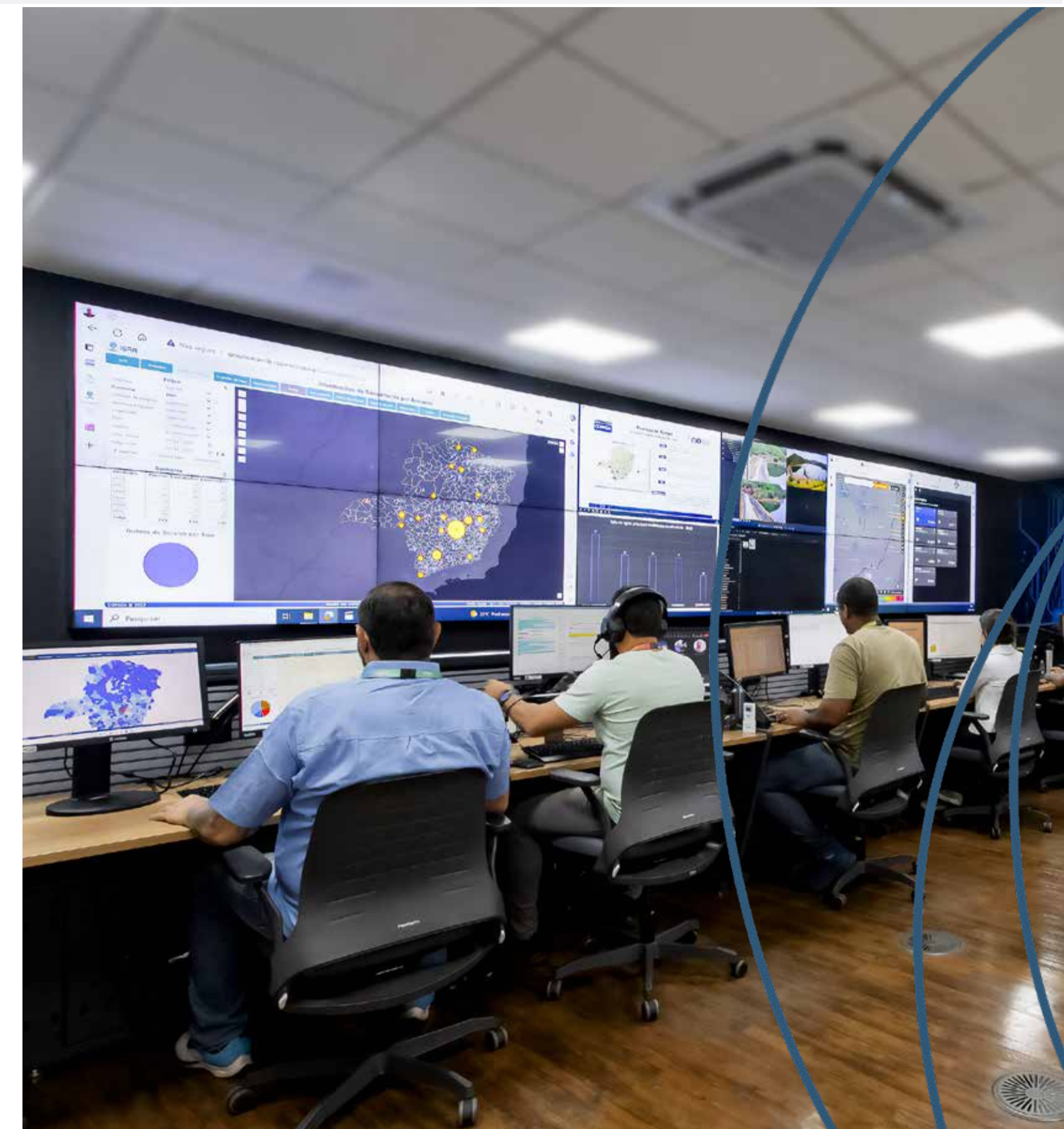
Copasa, COS Santo Antonio Control Room
