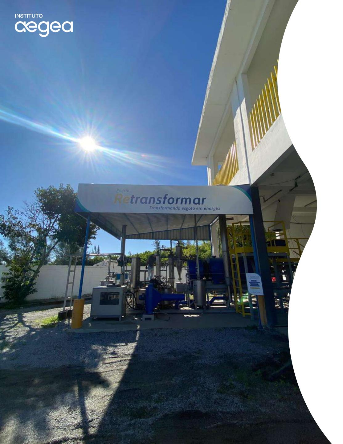
The Arraial do Cabo sewage treatment plant, owned by the Prolagos concessionaire, promotes the Retransformar (Retransform) Project, consisting of a pyrolysis plant that transforms sludge into biochar and synthesis gas, using 100% of the material. Furthermore, in 2023, 2377 tons (almost 100% of the total generated) of sludge from the WTP were reused, being sent to manufacture ceramics.
