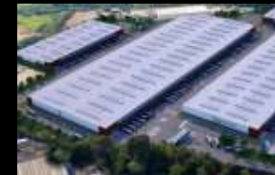
CLD (under construction) Warehouse São Paulo / 2023 128,516 sqm - total (17.03% SYN) 74,139 sqm - delivered
