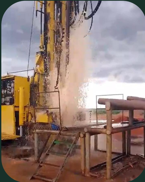
Well drilling 300m 3
