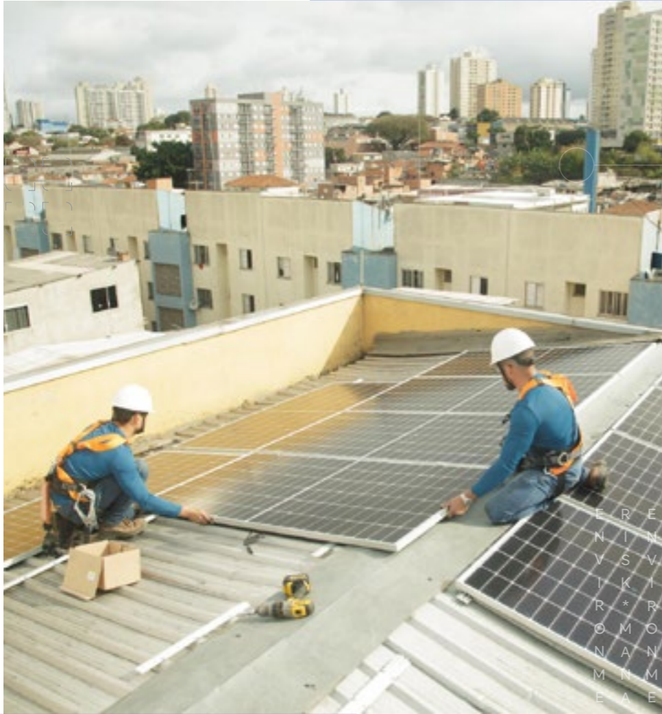
Installation of residential solar panels
