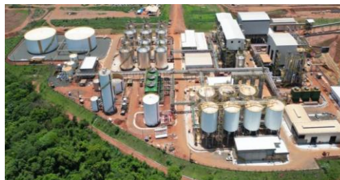
Plant #2 at Bonfim Bioenergy Park.
