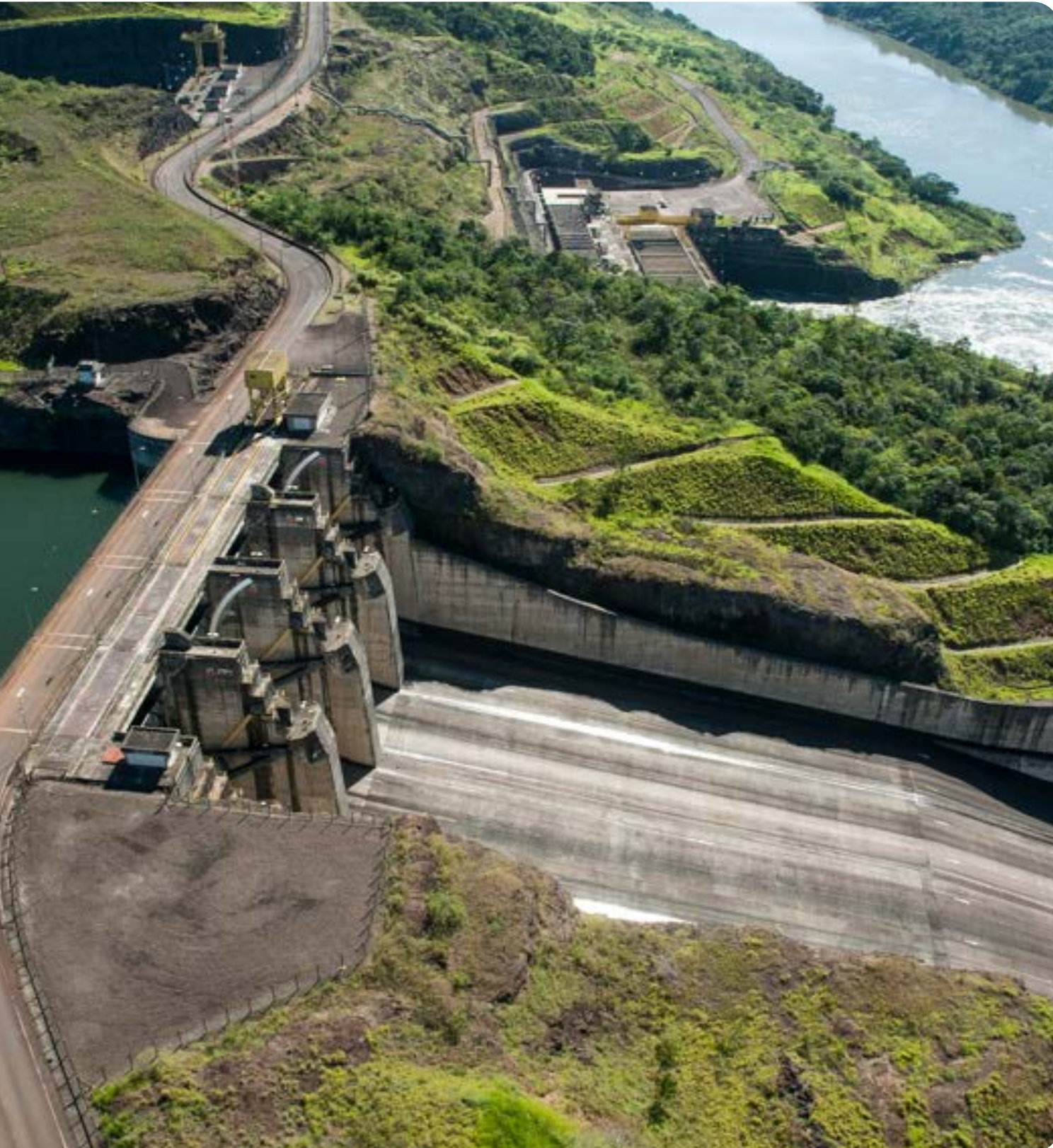
Itá Hydroelectric Power Plant (SC)
