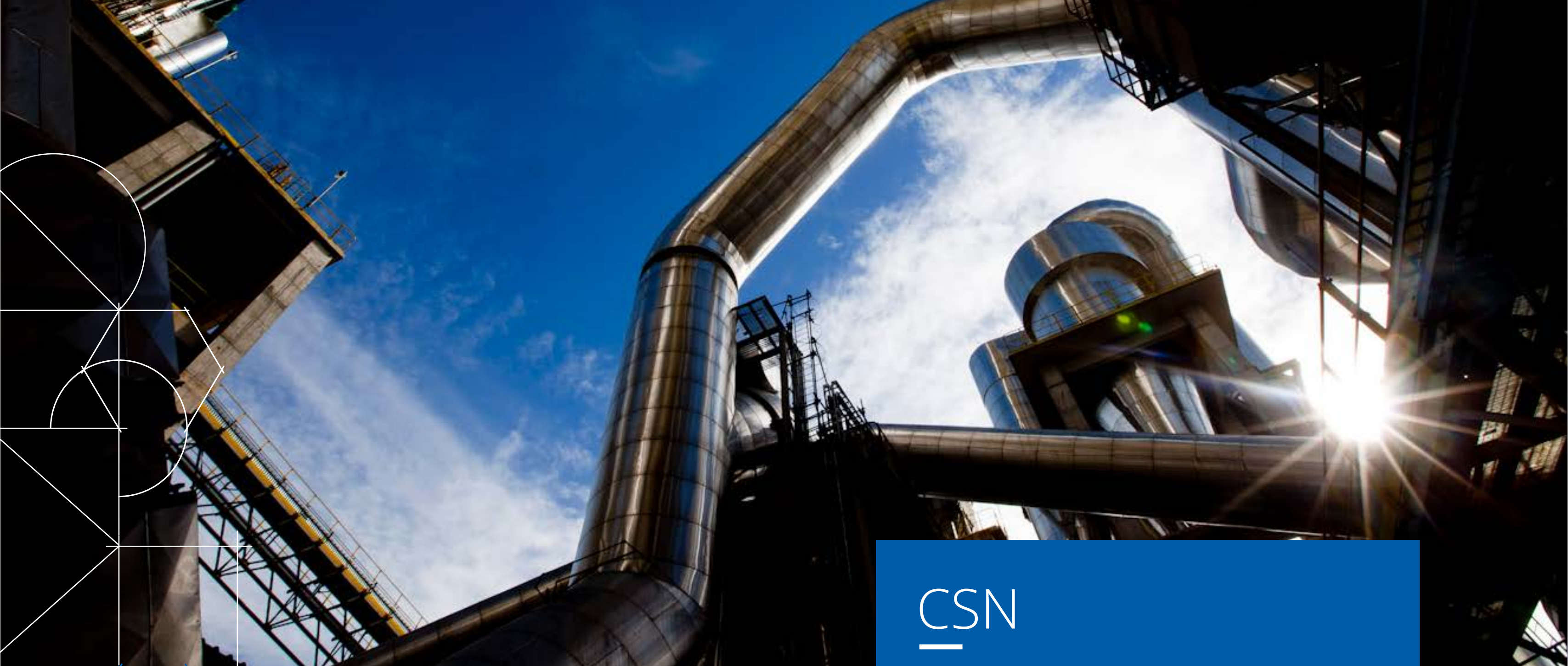
Cement Plant | Arcos (MG)
