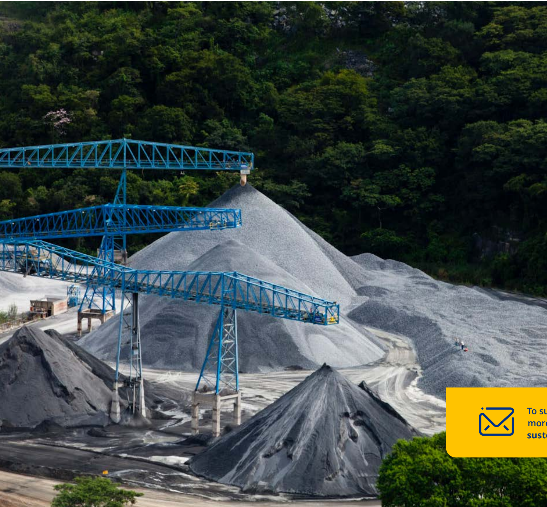
Cement Plant | Arcos (MG)
