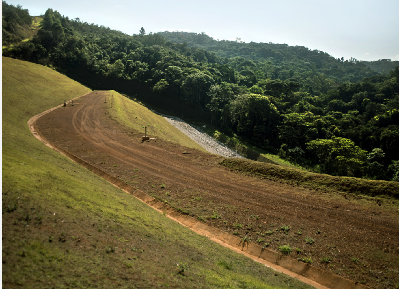
Left abutment of the saddle dike of the Casa de Pedra dam
