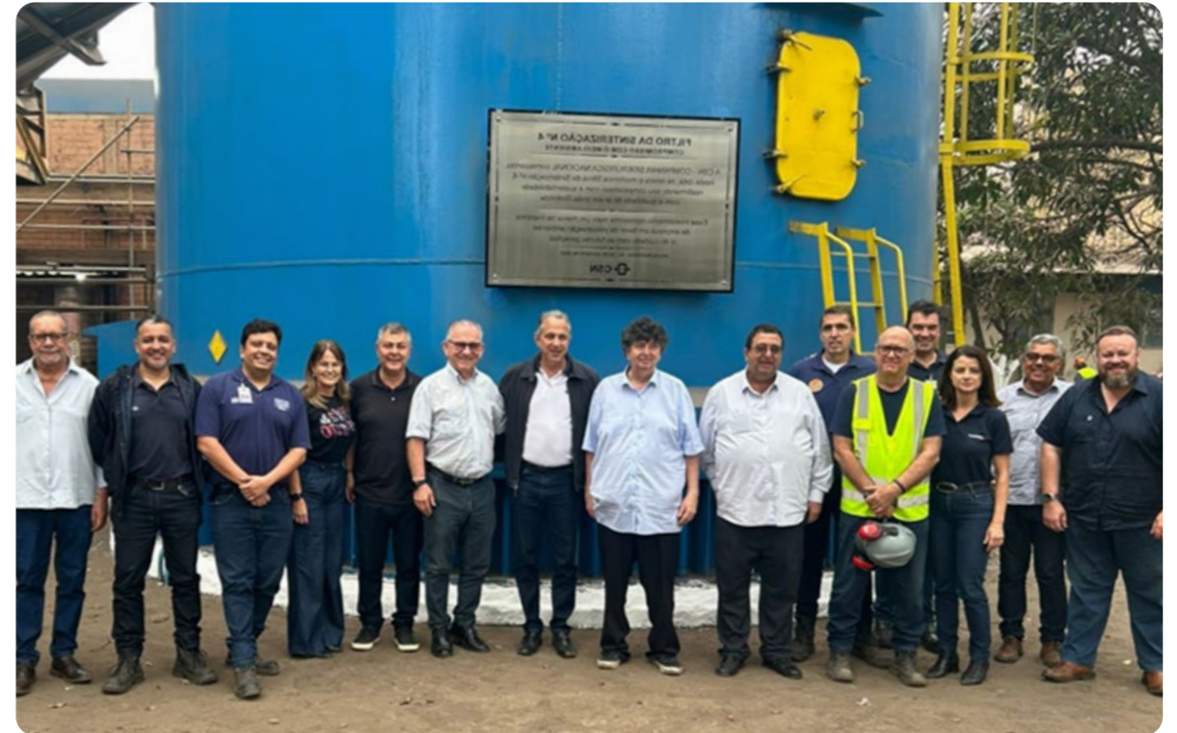
→ A new sintering plant environmental control system comes online – Volta Redonda (RJ)
