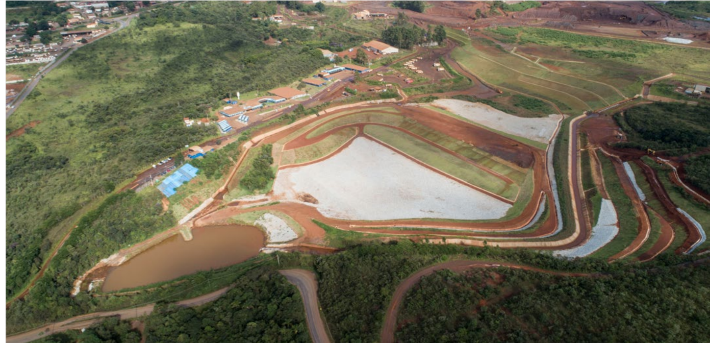
→ The Vigia and Vigia Auxiliar dams, both now fully decommissioned – Ouro Preto (MG)
