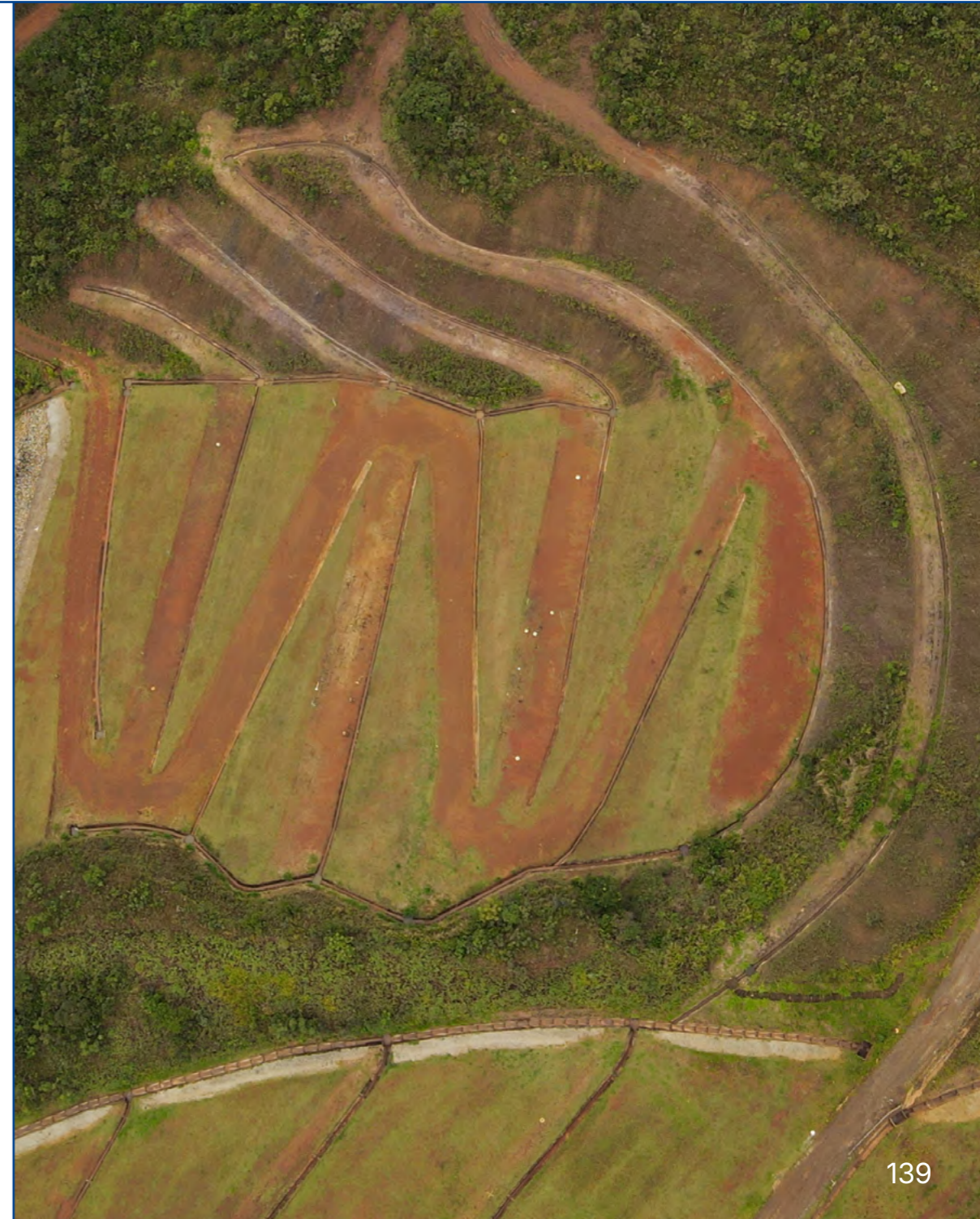
→ A saddle dike at the Casa de Pedra dam - Congonhas (MG)
