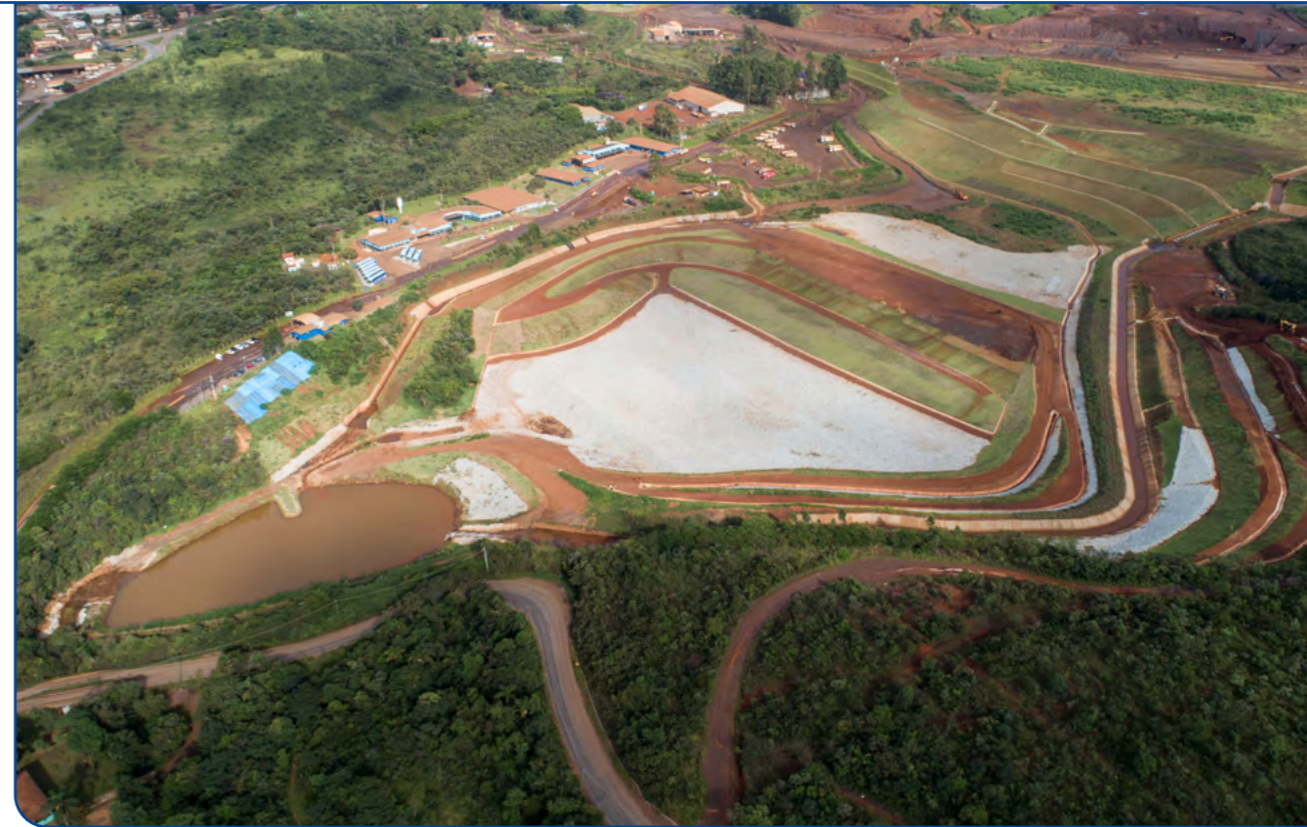
→ Aerial view of the Vigia Dam at CSN Mineração – Ouro Preto (MG)
