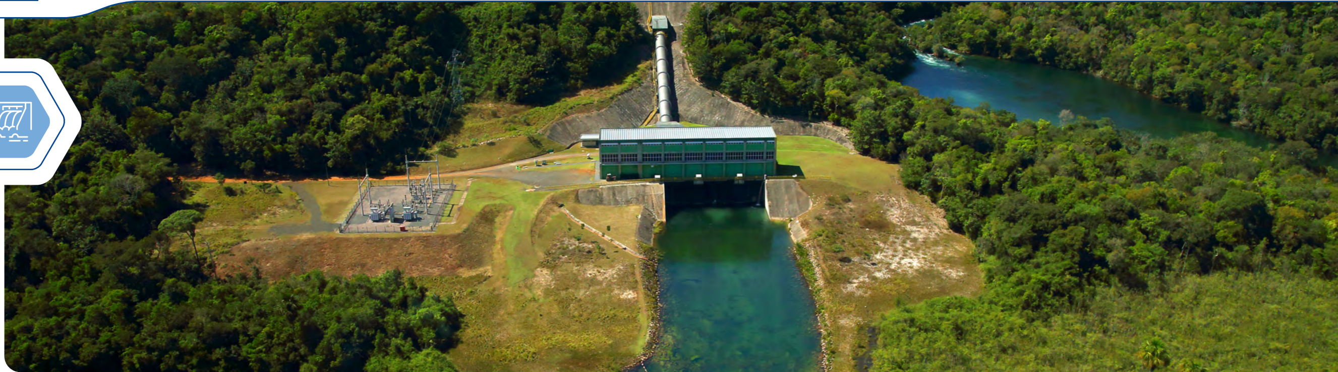
→ Aerial view of the Itá hydroelectric dam – Itá (SC)
