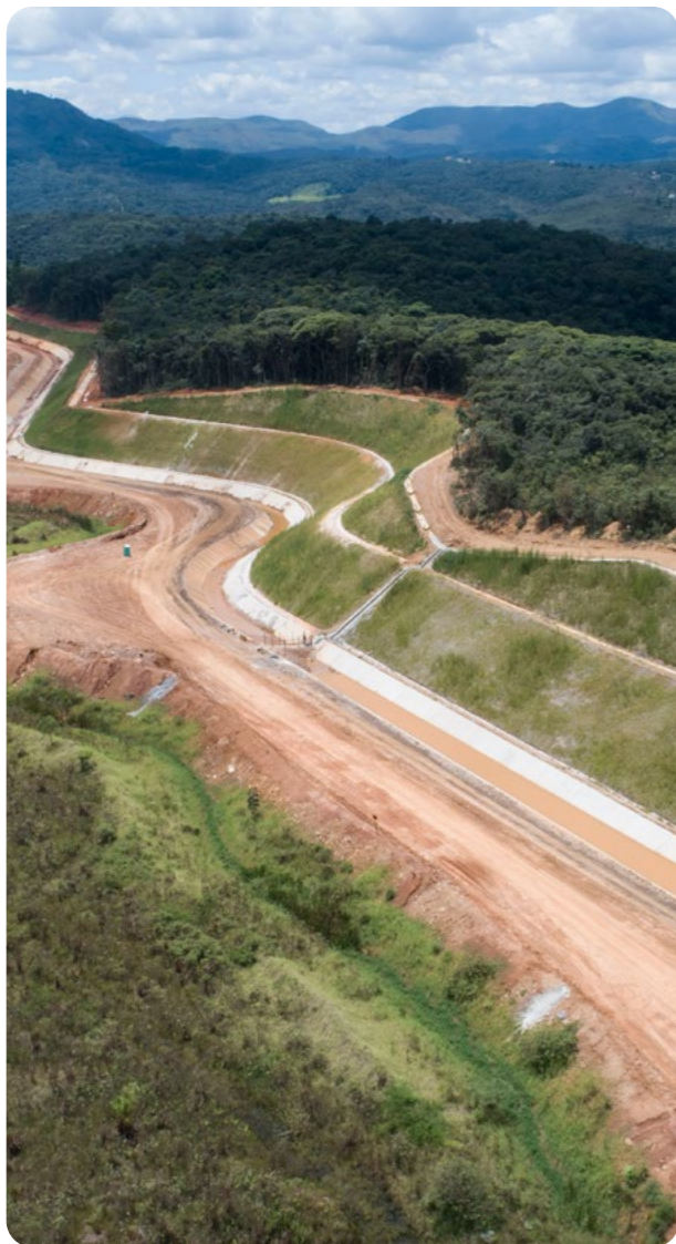
→ The B4 dam perimeter drainage channel - Congonhas (MG)
