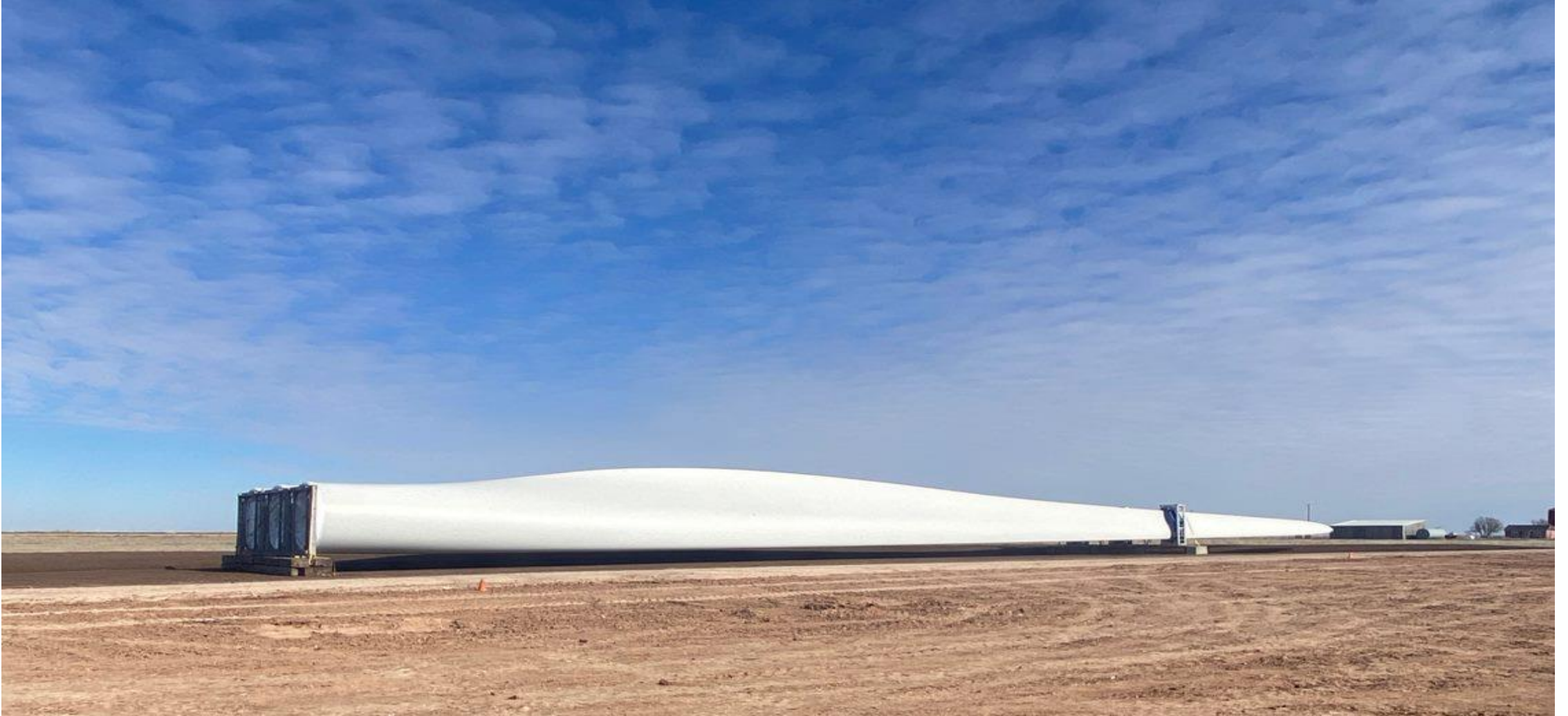
Goodnight 1: Wind blades being delivered on site.
