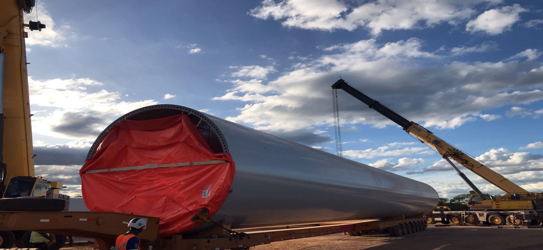
Assuruá 5: Components started being delivered for WTG assembly.
