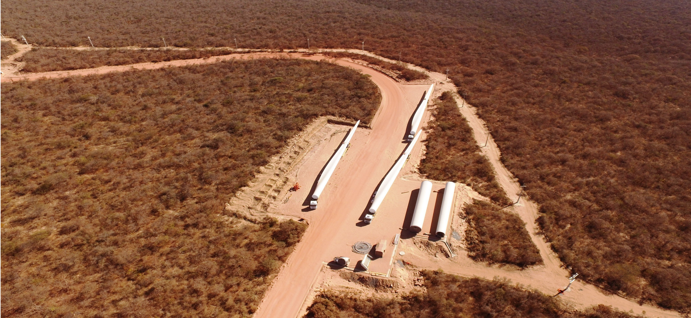
Assuruá 4: Main WTG componentes being delivered on site
