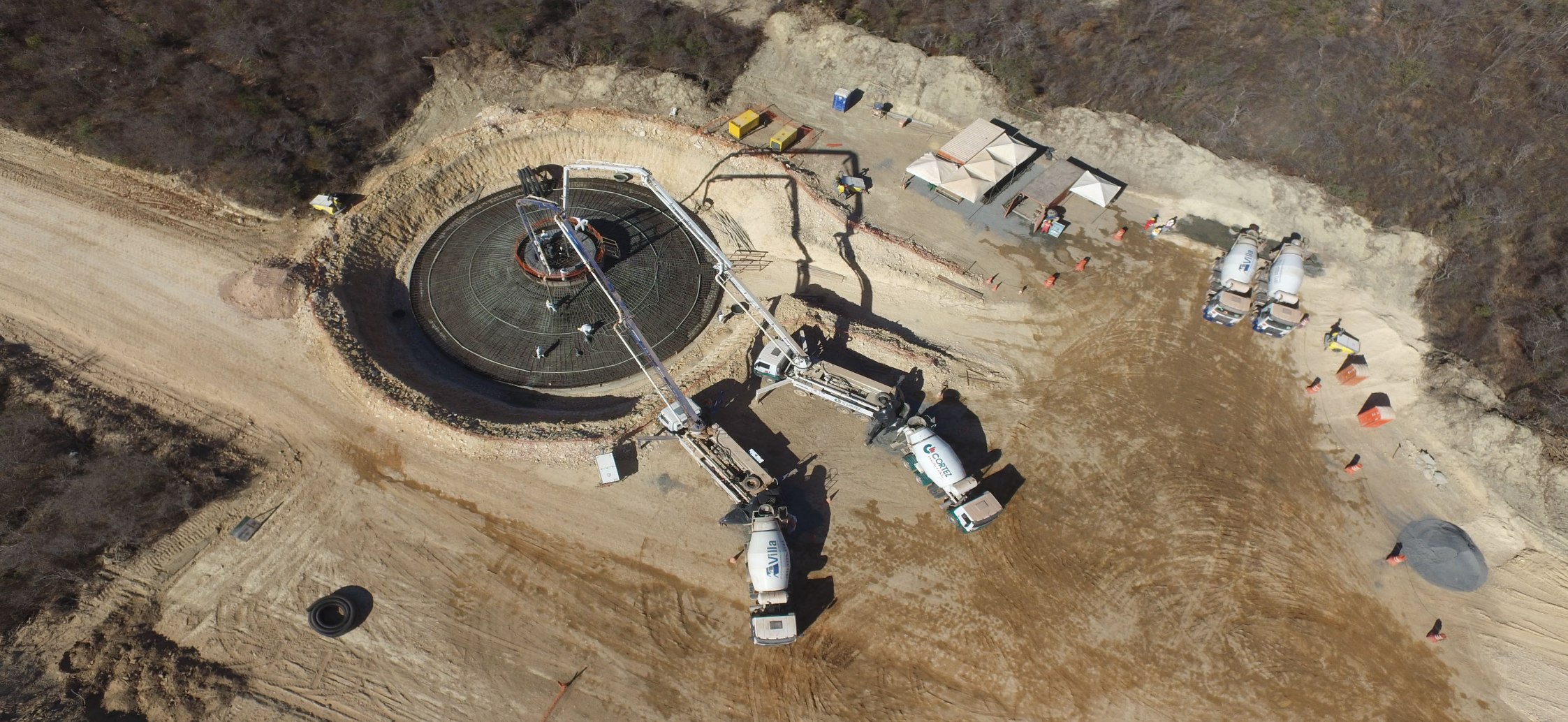
Assuruá 5 WTG Foundation (total of 42): 30 excavated and 18 framed
