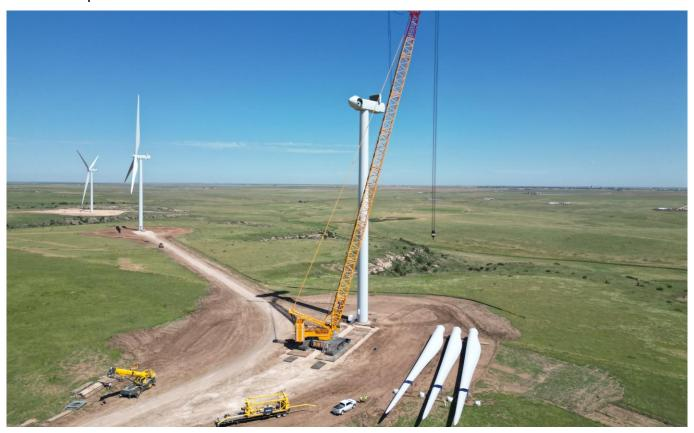
Turbine assembly has started and is currently in progress, with 3 out of 59 WTGs in mechanical completion.
