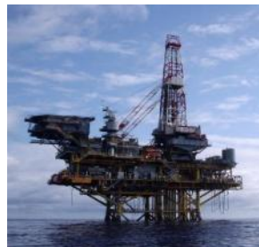
FIXED PLATFORM POLVO A
