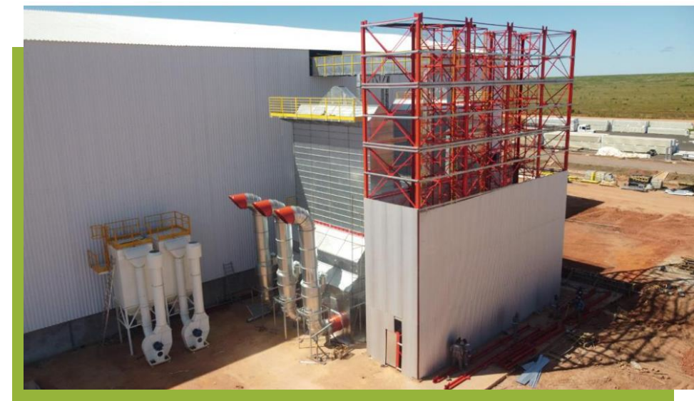
Construction in Progress
