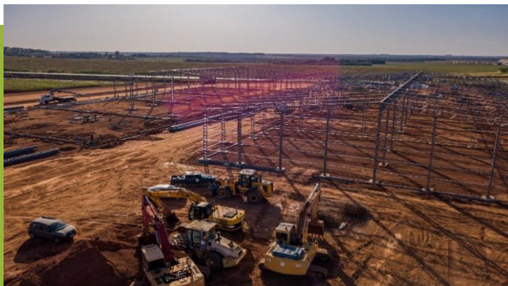
Beginning of works
