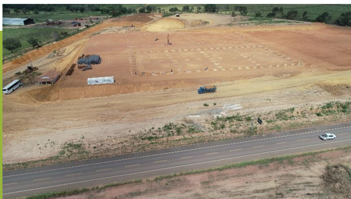
Beginning of works
