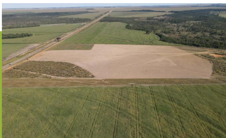
Beginning of works
