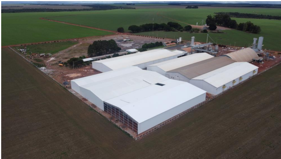
Construction in Progress / In Conclusion
