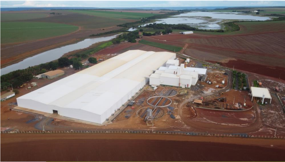
Construction in Progress / In Conclusion
