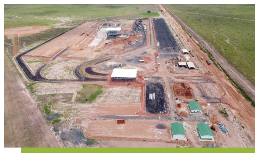
Constructions in Progress
